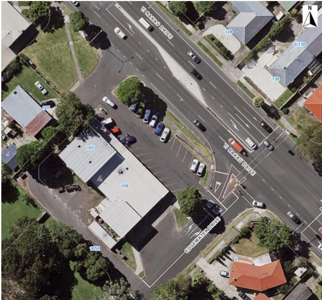
Figure 95: Edgewater Shops parking area
